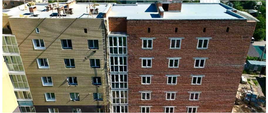
Restoring a residential building in Makariv, the Kyiv region
